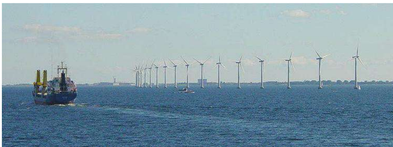
Figure 9.6. Offshore wind farm near Copenhagen (Denmark). Source: http://en.wikipedia.org/wiki/Offshore_wind_power
