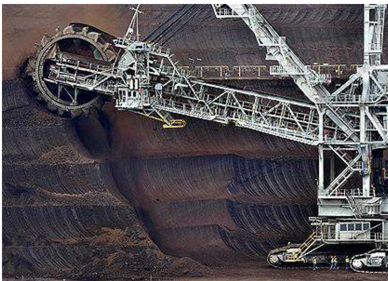
Figure 5.1. Open pit mine in Latrobe Valley, Australia, with an excavator. Source: http://www.theage.com.au/environment/brumbys-dirty-secret-coal-for-export-20091013-gvnp.html
