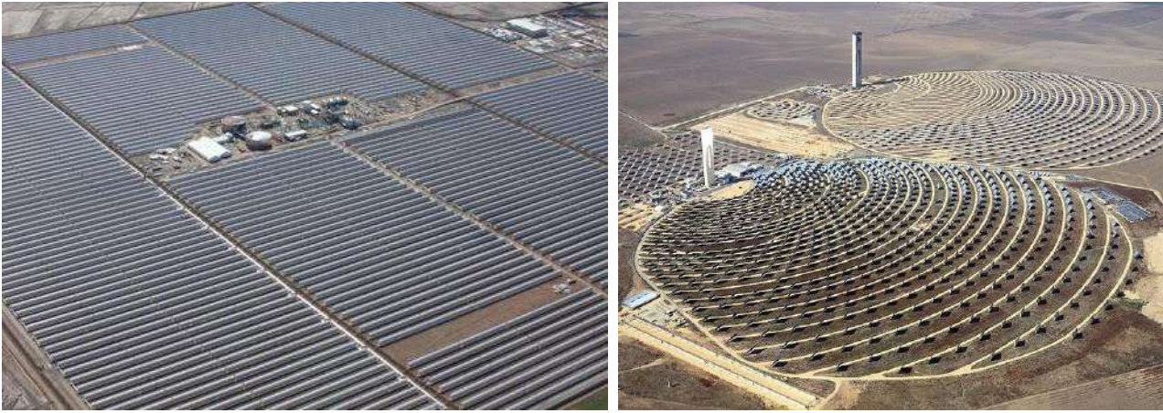
Figure 9.5. Solar thermal power stations. Left: Andasol I thermosolar park (Spain), with parabolic cylinder collectors and a thermal accumulation system by melted salts. Right: solar power tower plants, PS01, first, and PS02, second, with their corresponding heliostats (Spain)
