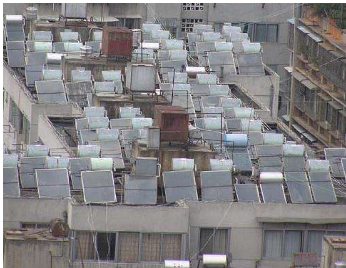
Figure 9.4. Hot water solar collectors in a Chinese city's roof
