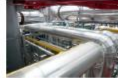
Combined heat & power
