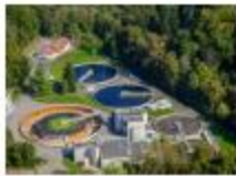
Water treatment & distribution
